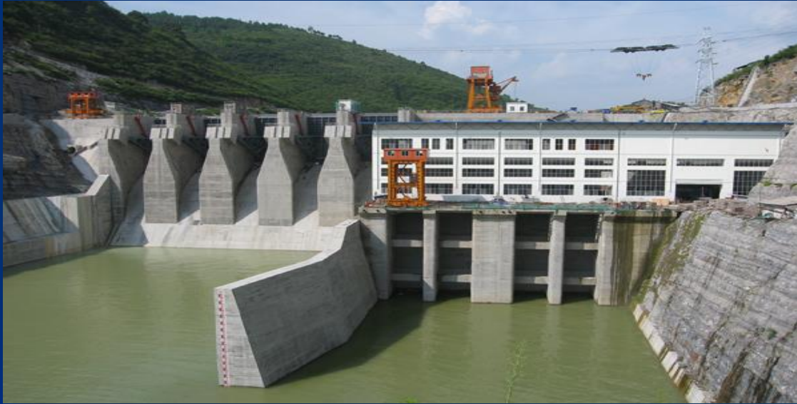
Video surveillance project of Hefeng Dam
